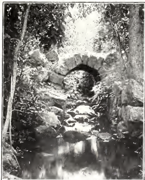
PLATE VI. AN HISTORIC MILL SITE.
